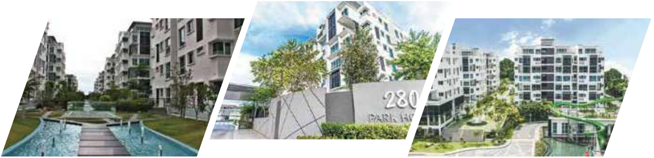
280 Park Homes, Puchong (Malaysia)
